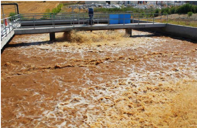
Aeration tank with surface aerators
