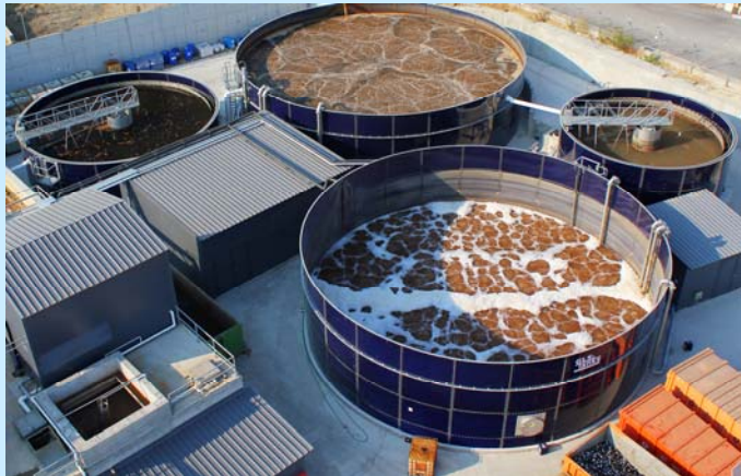
MBBR system - Prefabricated steel tanks.
