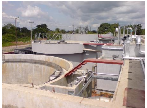
Sedimentation tanks
