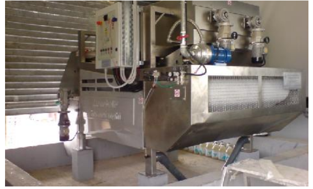
Sludge Dewatering - Belt Press
