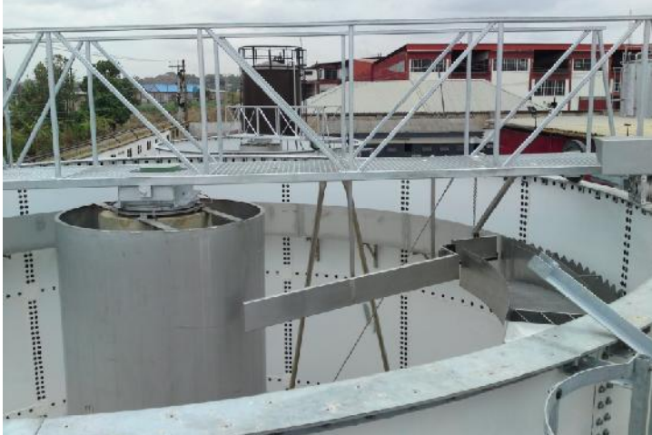
Sedimentation tank
