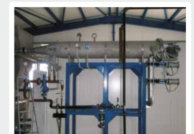
Combination of solids digestion with Rendering process for slaughterhouse by-products
