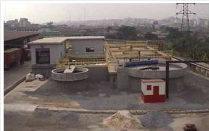
Activated Sludge Biological process
